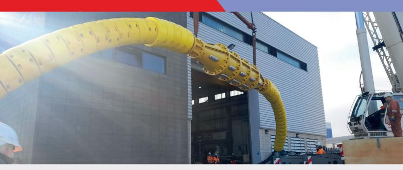
For the offshore repair of extra high voltage OWF subsea export cables (to 245kV) damaged during installation or operation Power CSL offers its innovative repair joint product.
